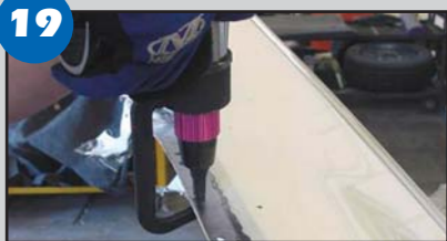
19 Drill out the remaining resistance spot welds for total access.
