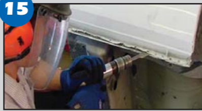
15 Separate the inner and outer panels with an air chisel.
