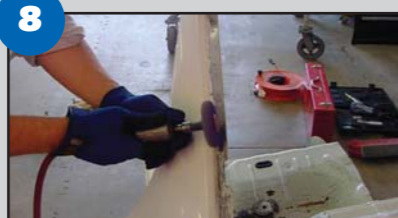
8 Remove the paint from the rear window pinchweld to expose the bare metal and resistance spot welds.
