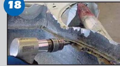
18 Separate the inner and outer wheelhouse panels with an air chisel.
