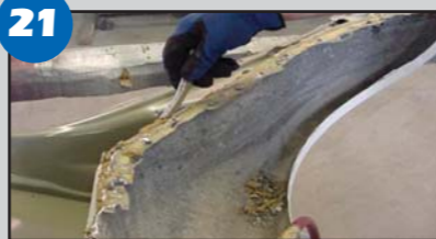
21 Remove all remaining sealant, adhesive and caulking.
